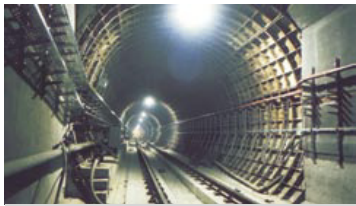
Fig. 2. Metro tunnel with cast-iron tubing
